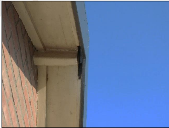
Fig. 1.16, Opening in nok (bron: FF Solutions)
